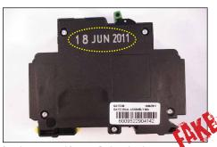
Date stamp on side of earth leakage device. Imitation devices have a machine applied mark, whereas authentic devices have 100% quality inspection and the date stamp is applied by a quality inspector by hand.
